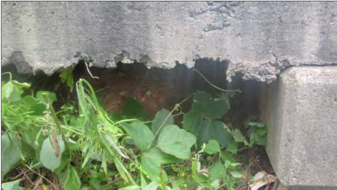
THERE IS A 3' LONG X 2' BACK AREA OF EROSION ON THE EAST APPROACH UNDER THE GUTTER AREA.
