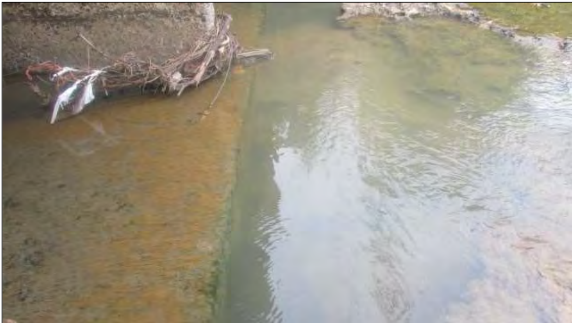
TOEWALL EXPOSED AT THE INLET. 1'X2'L AT BARREL 1 AND 3 AND 2'H X 3' L AT INLET OF BARREL 2.
