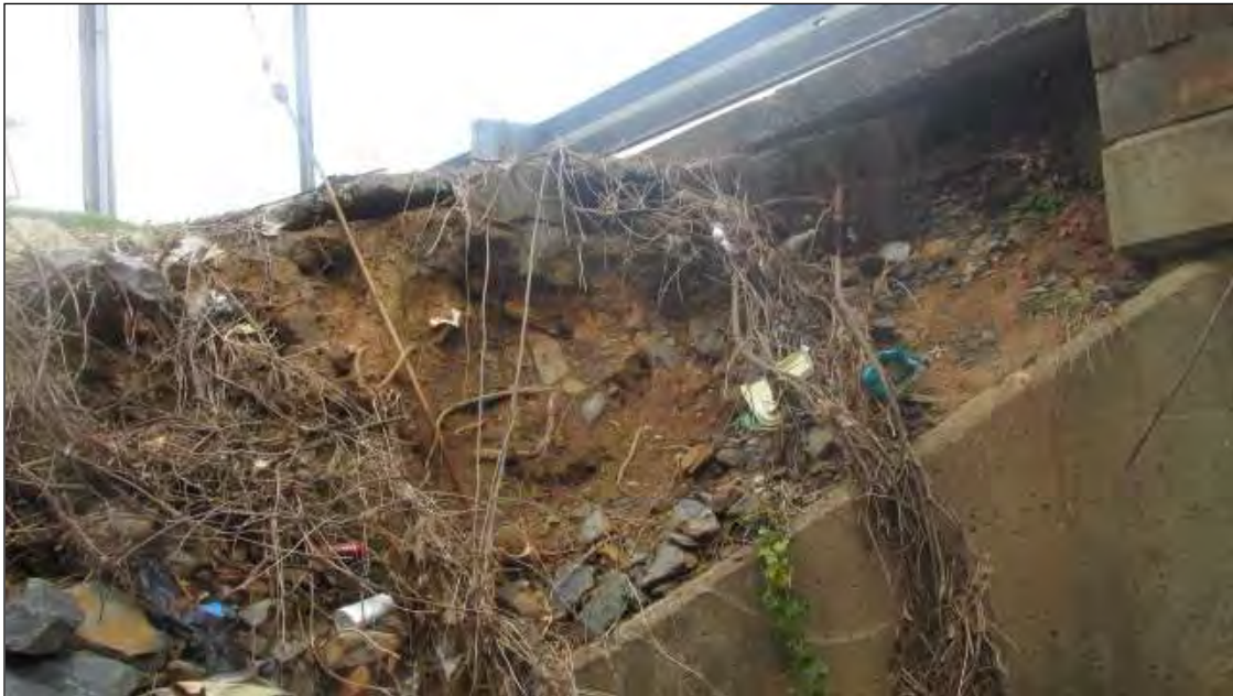
ERODED AREA AT THE SOUTHWEST CORNER BEHIND THE SOUTHWEST WING. EROSION IS 5'LONG X 4'W X 2'H.
